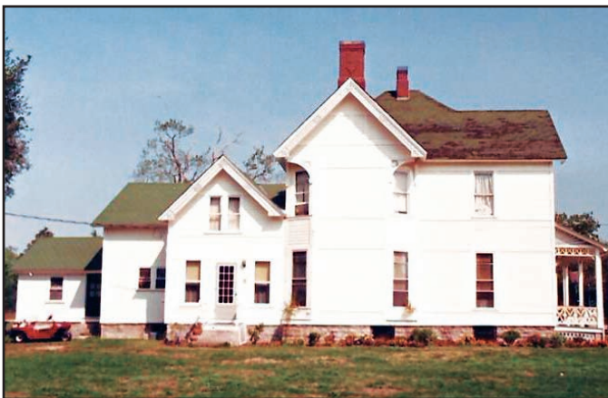
Before: Cameron House before it was lovingly restored by the Jorski Family.
