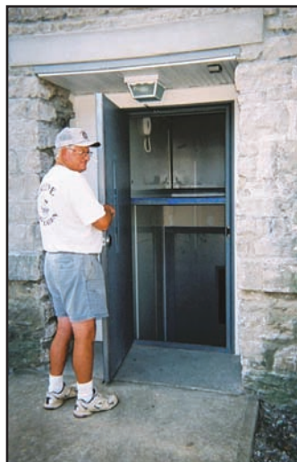
Photo by Carol Nelson-Burns Stan Greene installs new Town Hall elevator. It
