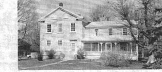
S-38 HISTORIC CENTURY HOME! Currently used as bed and breakfast; lake front lot with magnificent view. Ideal for the antique lover. Situated on 1 1/2 acres and included barn. Many bedrooms and a must to see!
