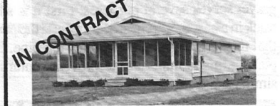
S-44 FULLY FURNISHED... and ready for your family. 2 bedroom and everything is almost new, inside and out. Back deck looks over lake. Enclosed front porch. Call now for more information.
