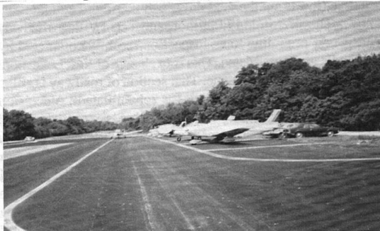
Newly paved plane parking area funded by runway widening grant.
