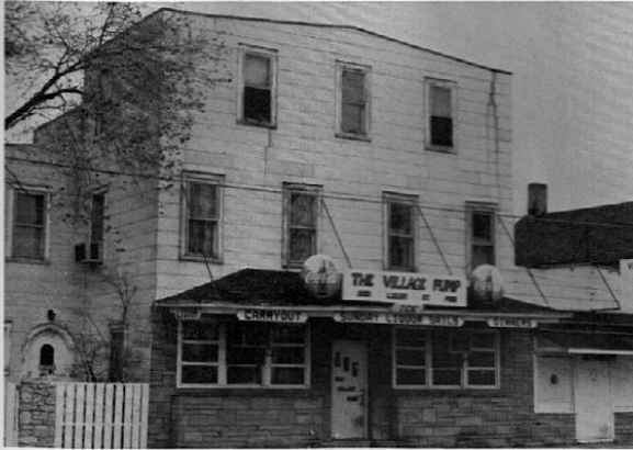
1. Village Pump - Built by Gus Kelley in 1890 as a combination barber shop and Post Office. The upper floor was used as a social hall.
