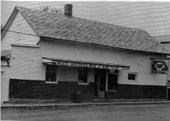
3. Island Market - Matso's Place and the Island Market were connected at one time. The building has been used as a library, United States Express Co. in 1885, and as a silent movie hall.
