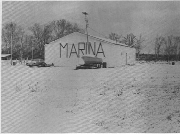
44. Marina - The Marina, once known as Kelley's Pond, was built in 1958. Many changes have taken place since then. The marina is a busy place in the summer. Small craft to large cruisers can be seen.
