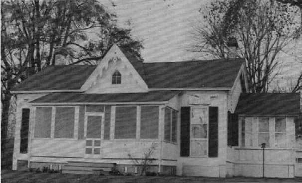
36. The Myers Home - This was the former home of Gus Son who was a well noted theatrical personality. The home is noted for its "gingerbread" affect trimming.
