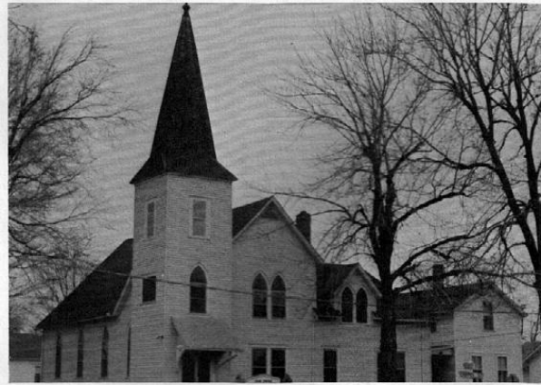
10. The Zion United Methodist Church - The church was started in 1893 and completed in 1894. The congregation consisted of 33 members. The altar was made from an organ of the Congregational Church which once stood across the street. Rev. Theodore Suhr was the first minister.
