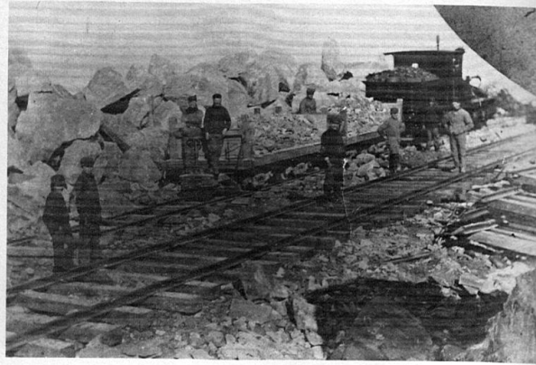
Quarry operation north side.
