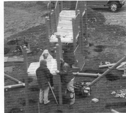
New playground equipment being installed.
