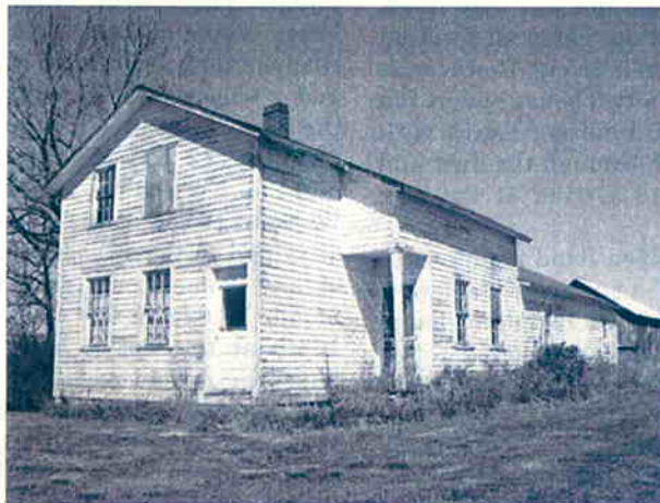
The former Kastning Home on the West side of the island (just past West Bay Inn).
