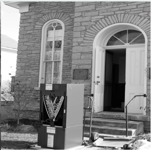
The heat pump and dehumidifier in Bayside Truck, the heat exchanger in front of the church, and (below) the passage to the south under the entrance stairway.
